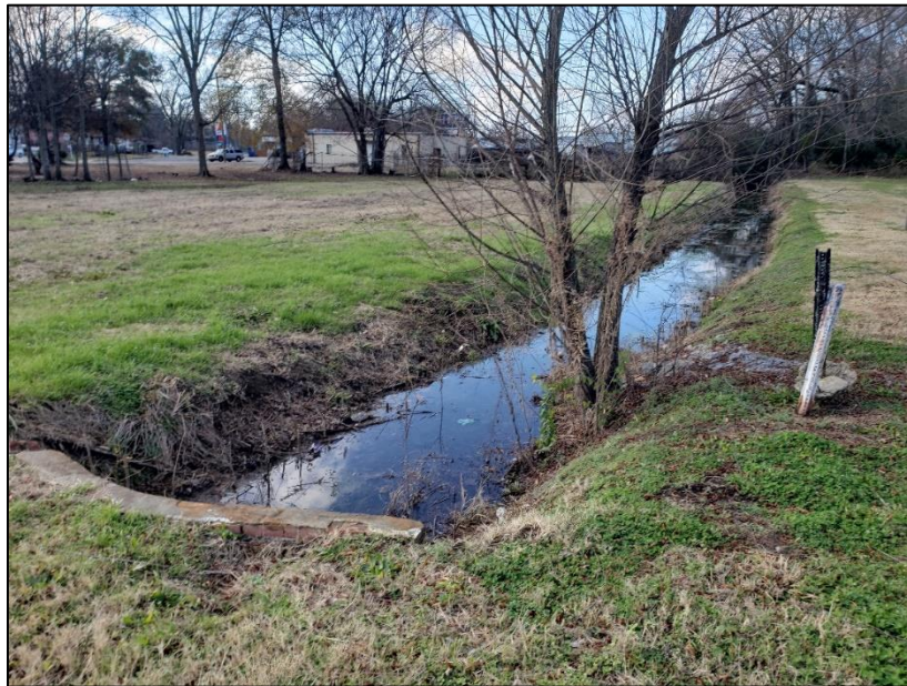
Figure 4-37: Drainage swale located between boring locations VD2-1-21 and VD2-10-21.
